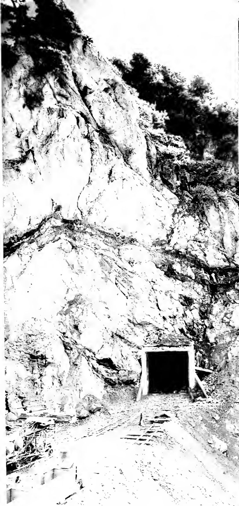
At left, portal of tunnel No. 2 through ridge of Mt. Williamson. This is a 14 x 14 foot pilot bore. At right, top, equipment mucking at main heading of tunnel No. 1, showing protective shell in use. Below, Construction yard between tunnels. Building concrete tunnel lining form. In the background may be seen the portal of tunnel No. 1.
